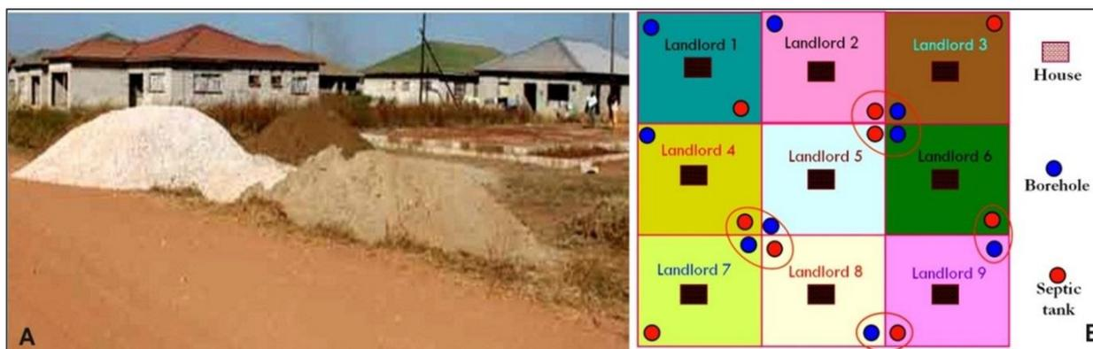
**Figure 8. (A) Construction of Houses in New Settlements, and (B) Envisaged Configuration of Boreholes and Septic Tanks for Each Dwelling in Lusaka's New Low-Density Settlements.**
