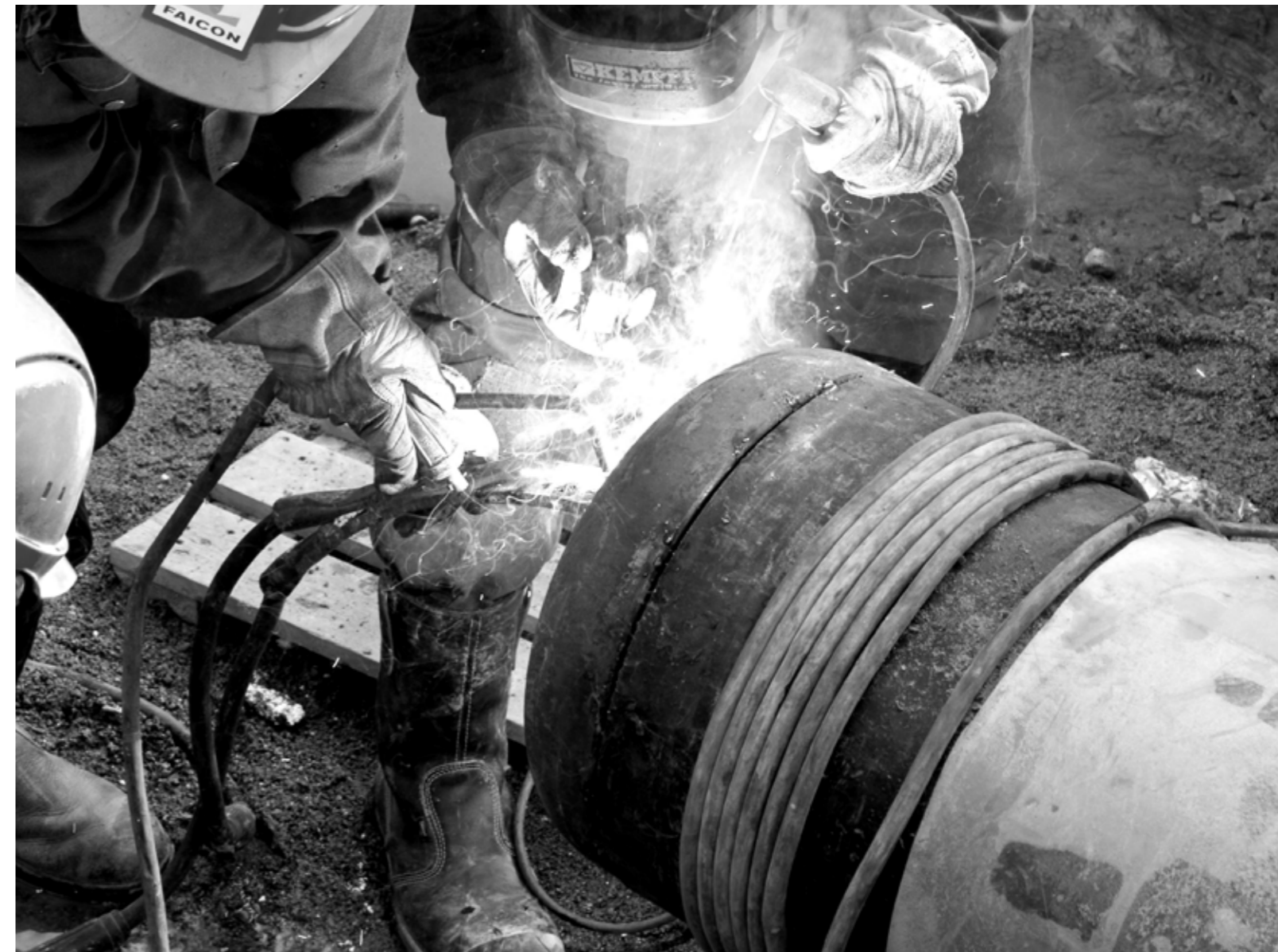
Construction of a natural gas pipeline Photo Credit: Gasum Oy
